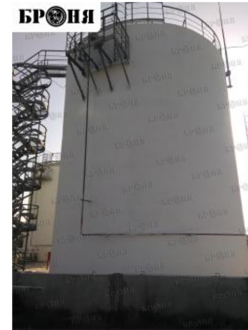
Thermal insulation and corrosion protection of the reservoir enclosures using Bronya liquid heat insulating materials:
